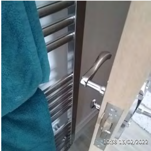
81 Bathroom trade Carpenter Door stop required
