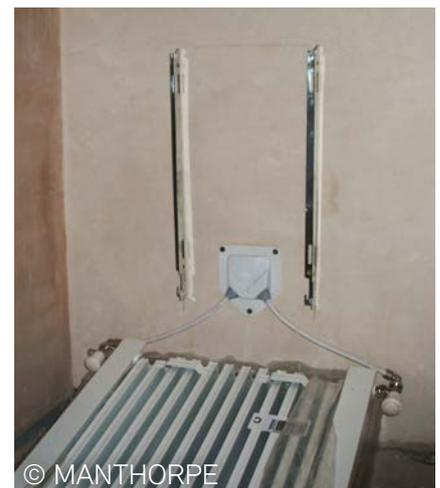
RADIATOR SEAL SOLUTIONS - INSTALLED SEAL
