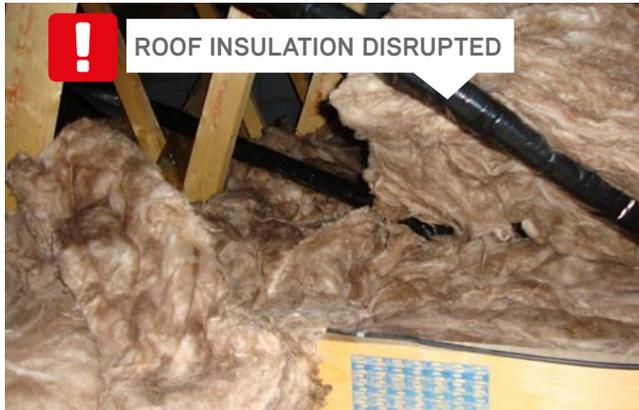
POOR PIPE SUPPORT DISRUPTS INSULATION IN ROOF
