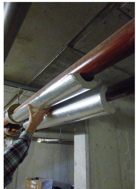
ADEQUATE INSULATION AROUND PIPES IN CORRIDORS AND FLATS
