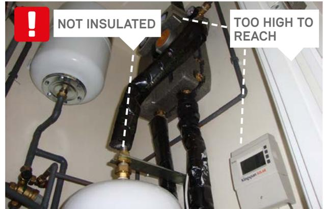
PARTIALLY INSULATED SOLAR PIPEWORK AND INACCESSIBLE CONTROLS
