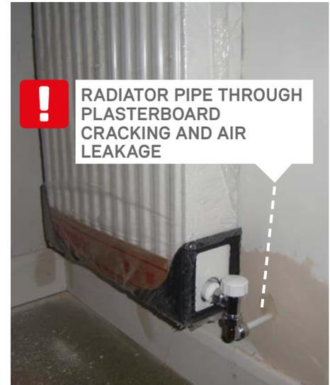
AIR LEAKAGE TO OUTSIDE AND UNDERSIZED RADIATOR
