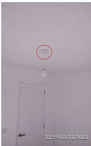
Rear Bedroom Right Assigned To Building Contractor The ceiling rose is loose fitting
