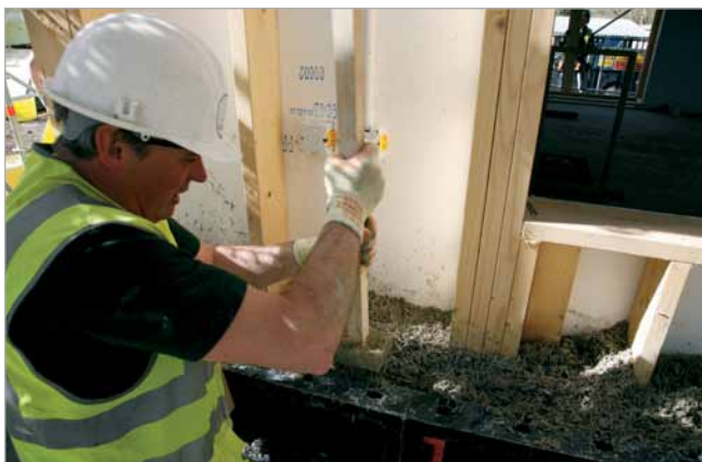
Hempcrete house during construction
