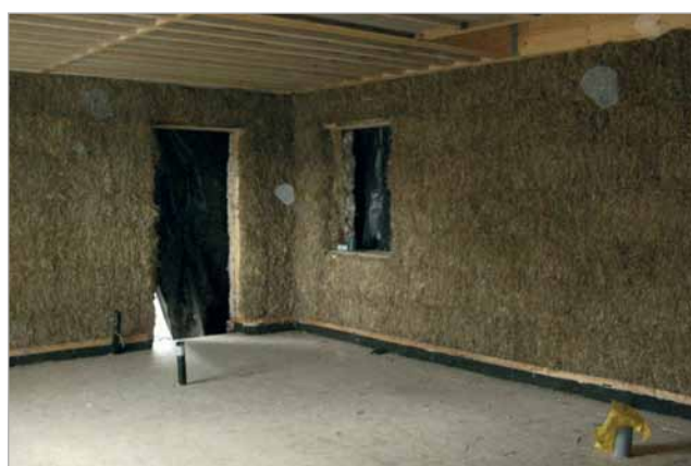
Straw bale house during construction
