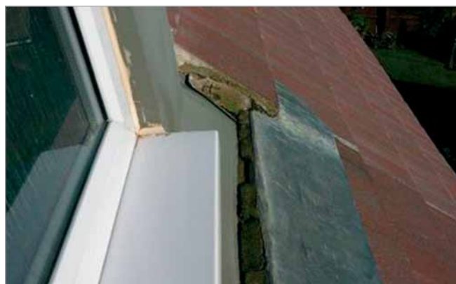
Unsuitable detail leading to mortar failure and water ingress
