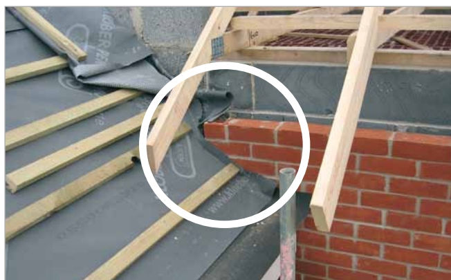
Underlay cut too short to form adequate lap when flashing is introduced
