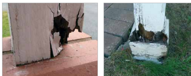
Examples of porch post failures
