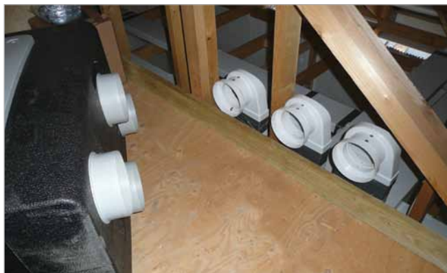
MVHR system being installed
